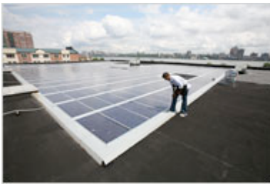
A Whole Foods store in New Jersey has solar panels.
